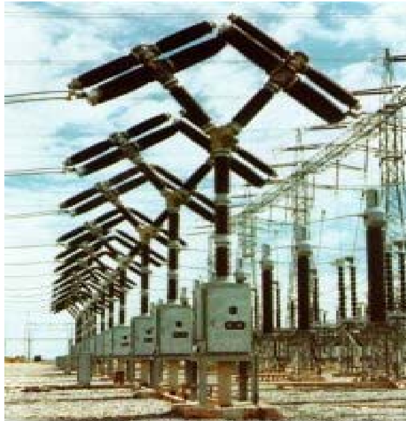
550kV (BIL 2100kV) SF6 GCB (equivalent to 800kV GCBs)
